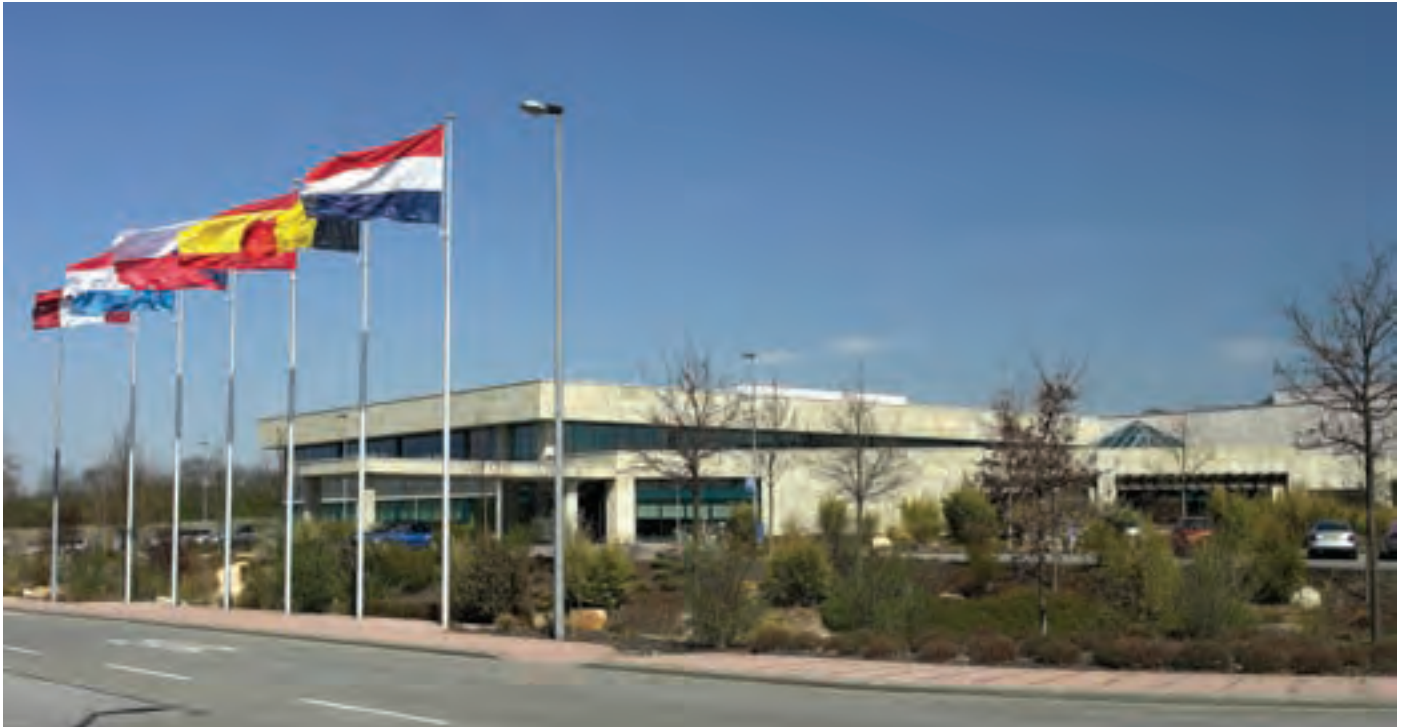
Husky Luxembourg facility
